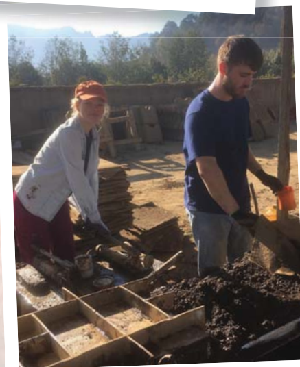
Team members from Robinhood Road Baptist in Winston-Salem make adobe block on-site. This process is vital to the ministry of the Good Shepherd in Xela.
