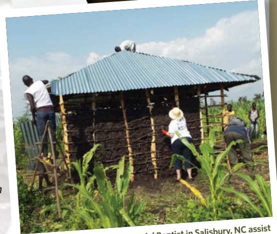
The team from Stallings Memorial Baptist in Salisbury, NC assist in putting matopi (mud) in the chinks of a new Kenyan House of Hope.
